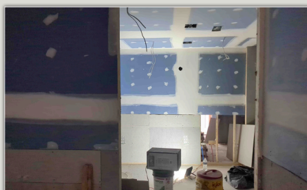
With the framing and sheetrock complete, the walls are ready to be painted.
