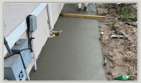
A concrete slab has been poured. Moving forward with construction!
