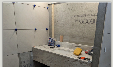
Ceramic work moves forward at full speed.
