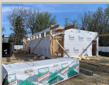
Framing the outer walls of the mikvah building
