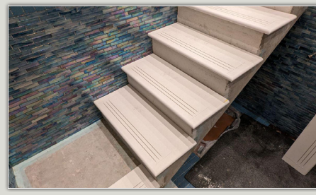
Next step! Tiles are installed on the steps of the Bor Tevillah.
