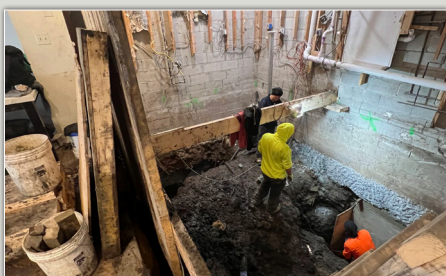
Ongoing demolition work to replace the old building with a gorgeous new mikvah
