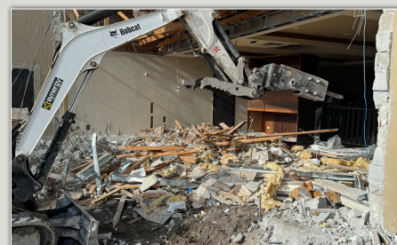
Full speed ahead! Demolishing the old building to make room for the new
