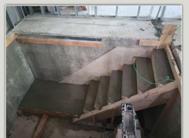
Getting there step by step. Laying the concrete for the steps in the Bor Tevillah
